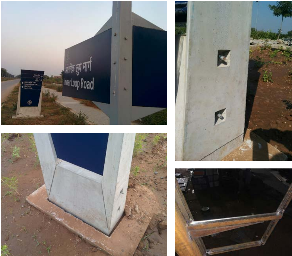
Figure 41. Construction techniques for concrete and aluminium structures
