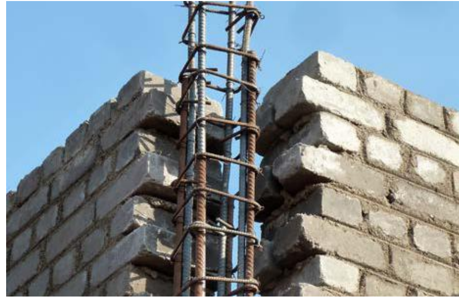
Locally sourced fly ash was used to manufacture the FALG (fly ash) bricks on site
