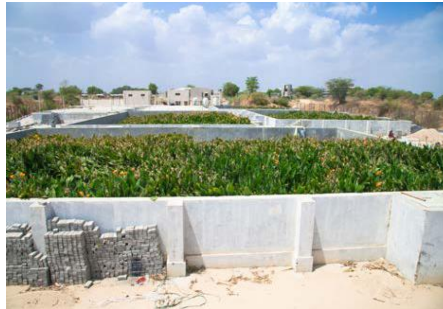
Root Zone Treatment system, where Canna indica plant roots absorb pollutants from effluent, as part of sewage treatment process
